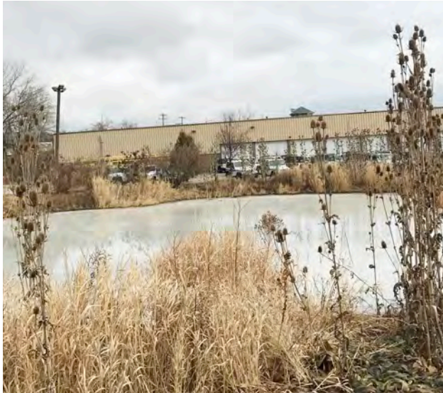
View of retention pond with building behind
