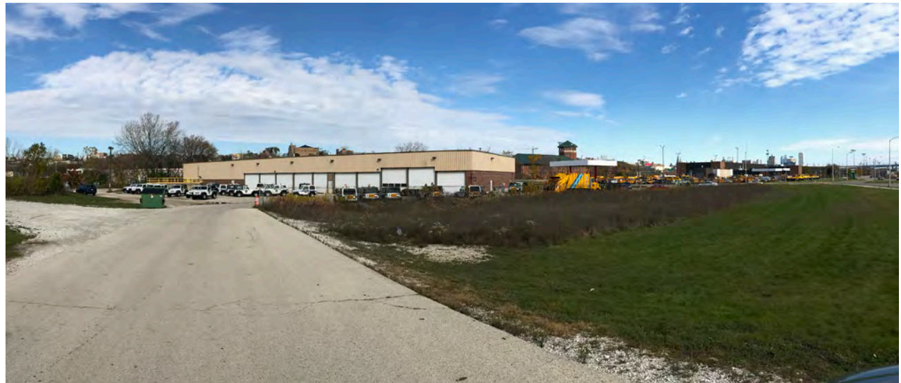
View looking at building and right-of-way
