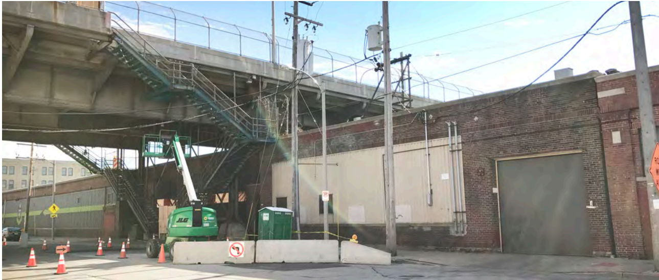
Connection from St. Paul to 16th Street, 1601-1539 W St. Paul Ave.
