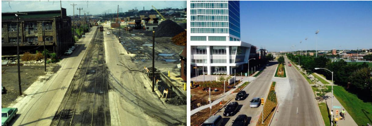
Images 1 and 2: Canal Street looking west from the 16 th Street viaduct, 1980s (left) and today (right)
