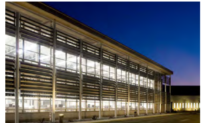
exterior glazed facade
