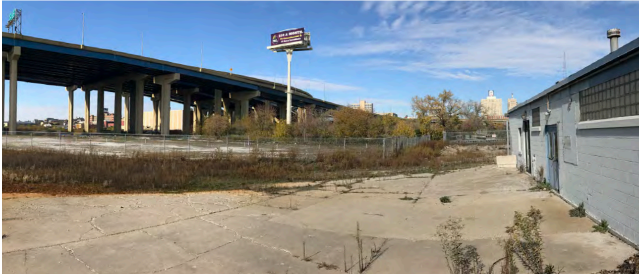
View looking northwest at riverfront edge and interstate
