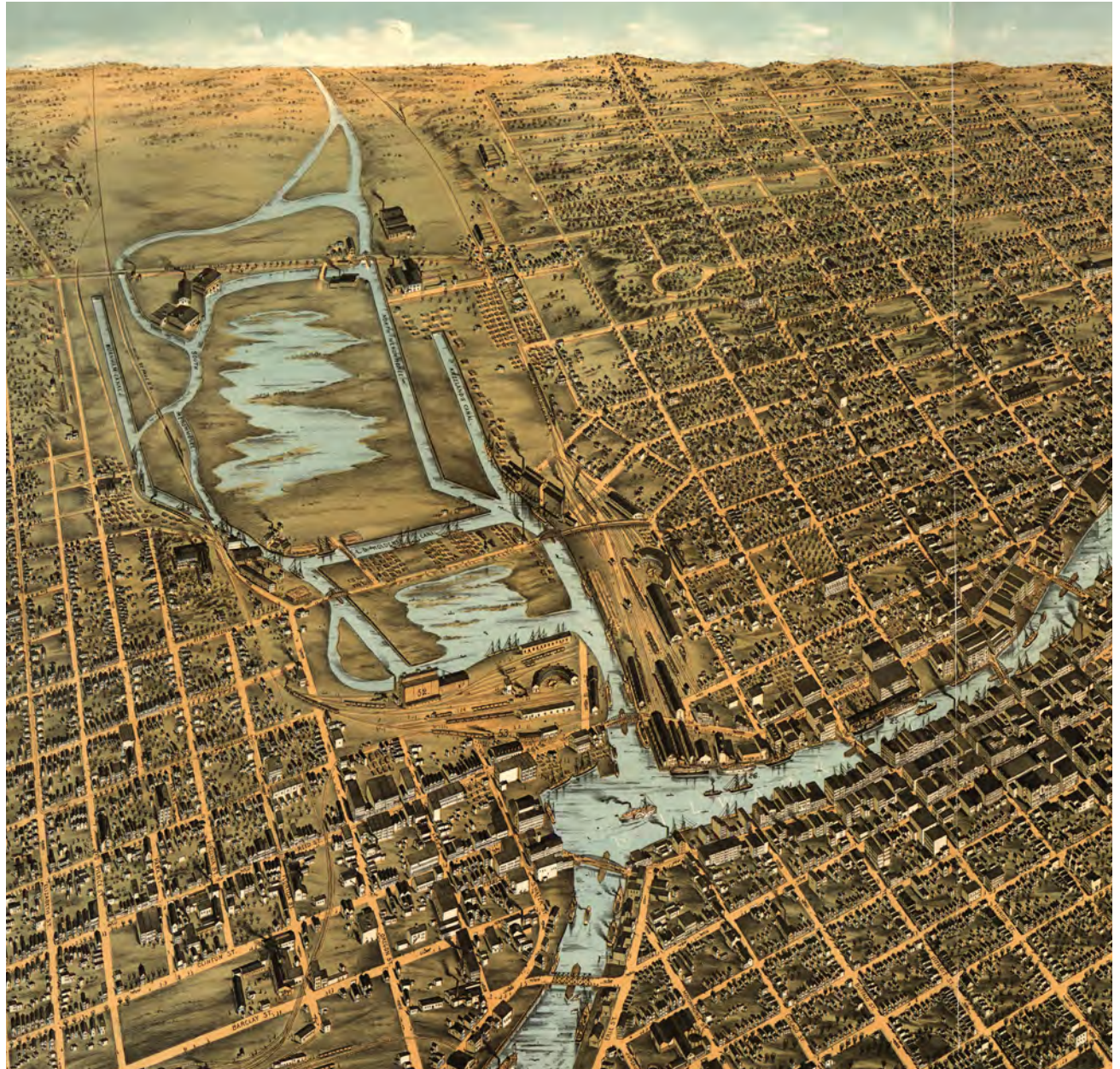
View looking west across the Valley source: www.renewthevalley.org
