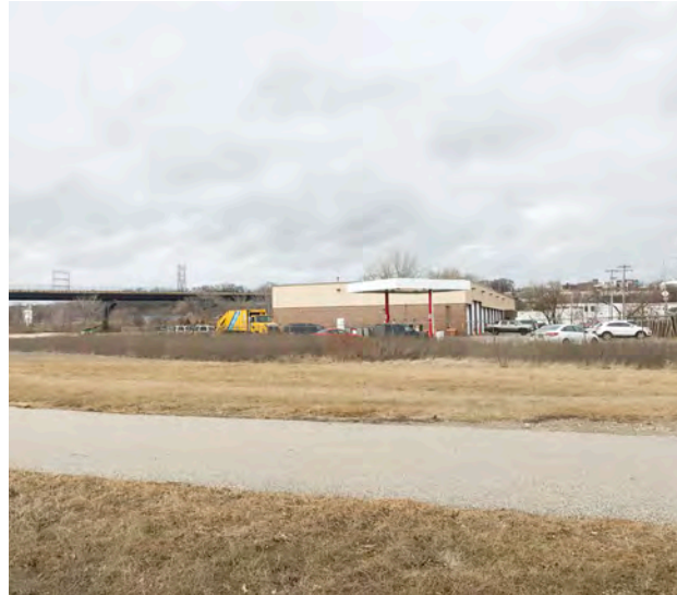
View of building from Canal St.
