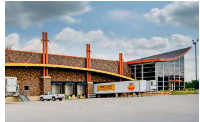
exterior view of the loading dock
