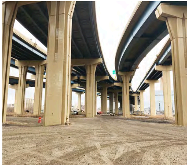
View looking south underneath the interstate
