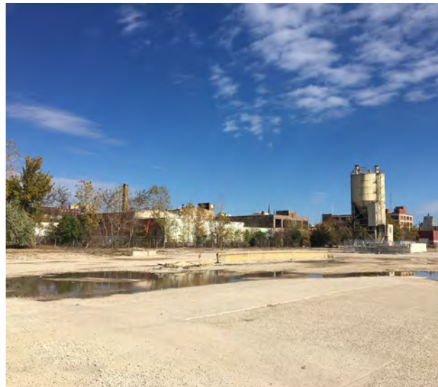
View of northern edge of site
