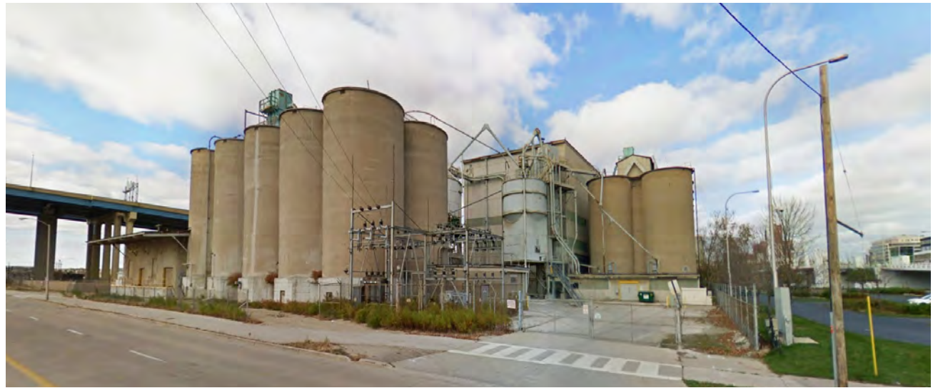
View of the silos from Canal Street
