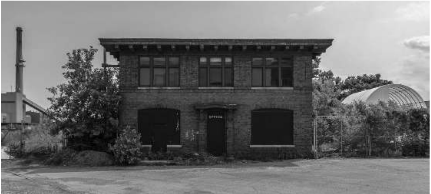
Figure 1.02 - Historic Office Building
