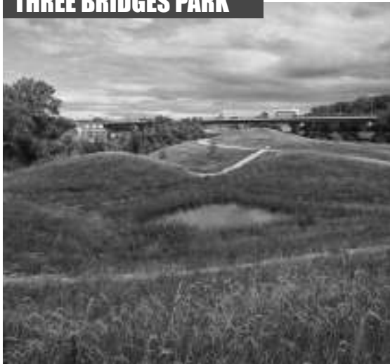
Figure 3.07 - Three Bridges Park Site Photo
