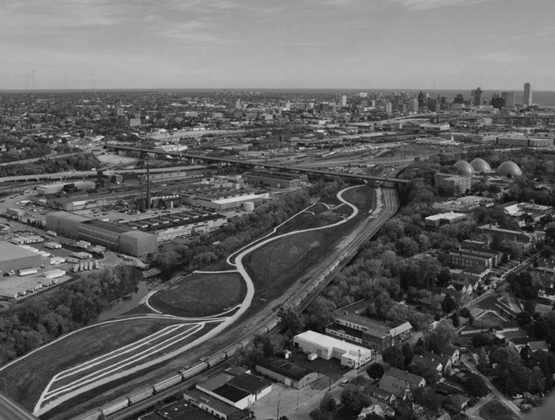
Figure 9.01 – Three Bridges Park Aerial Photo
