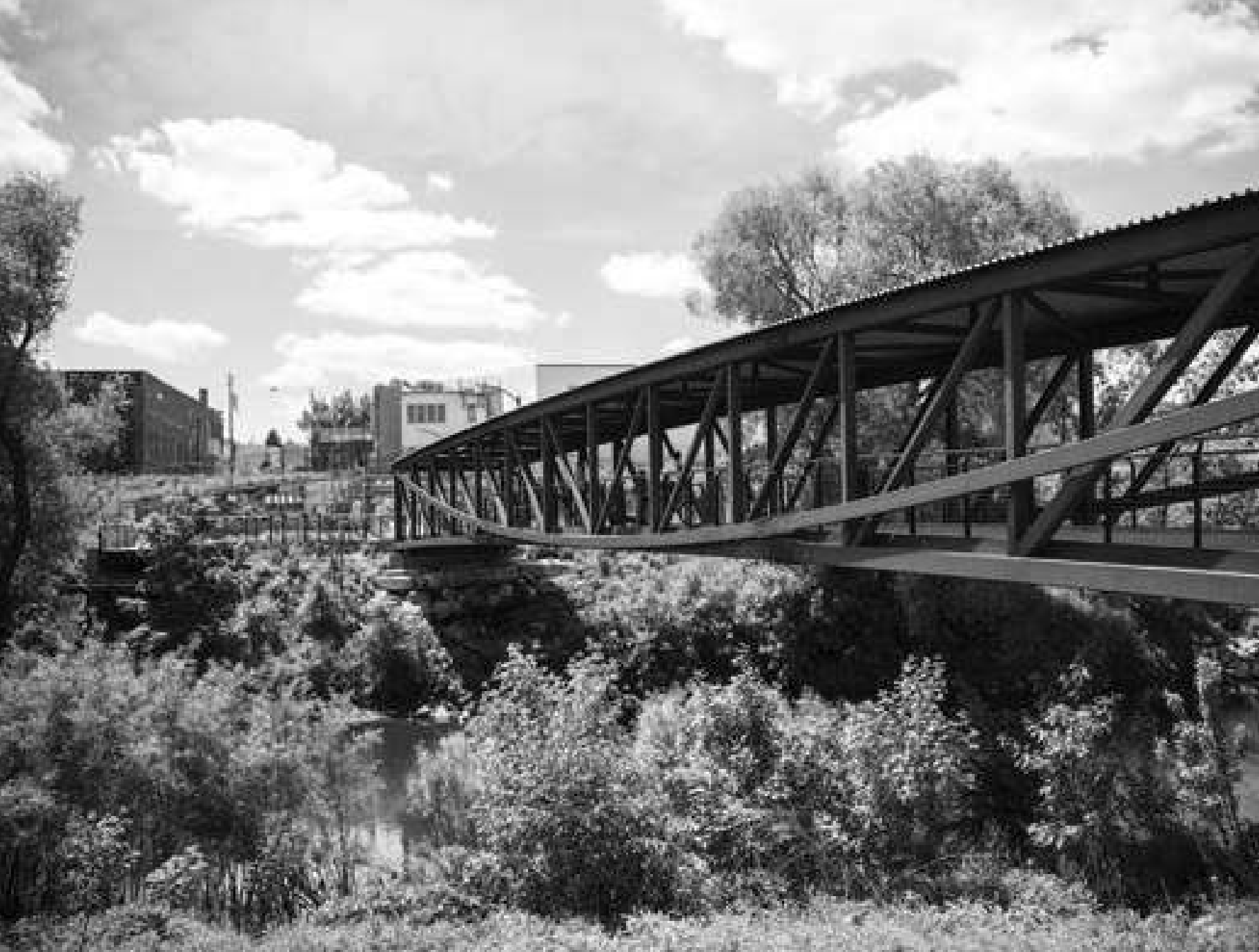
Figure 10.01 - Hank Aaron State Trail Bridge
