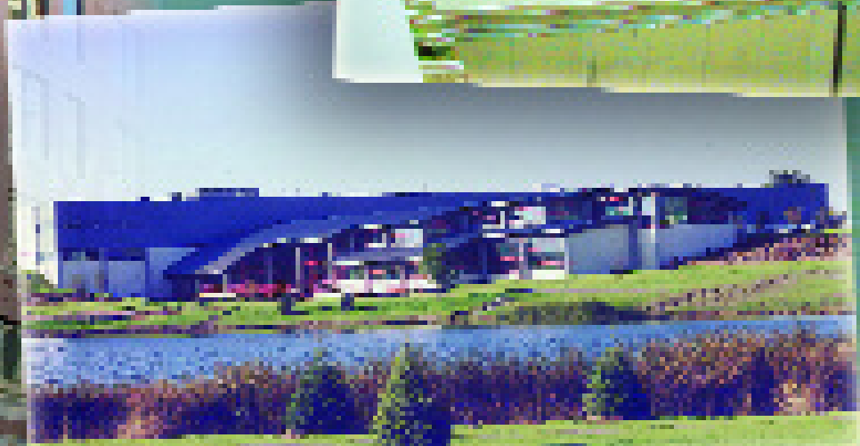
Office and factory workers share common amenities in the Danfoss Fluid Power Factory and Headquarters (Racine). The manufacturing plant is filled with natural light from rooftop monitors, fresh air ducted to the factory floor and views to the exterior. The office portion was designed using a glue-laminated wood structure, natural ventilation and daylight throughout and low-emissivity interior finishes.
