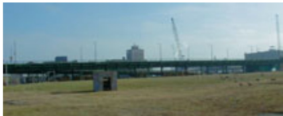
Current view (1999) of the 6th Street Viaduct spanning the East Valley.
