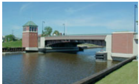
The new Ember Lane bridge at 13th and Canal Streets.
